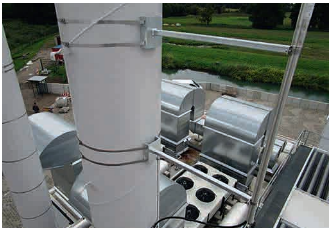
Spacer with tensing strap fastener
